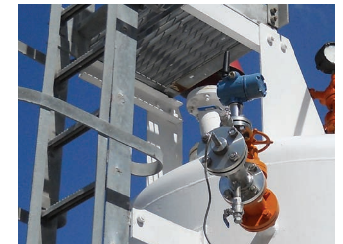
Rosemount 2160 installation
